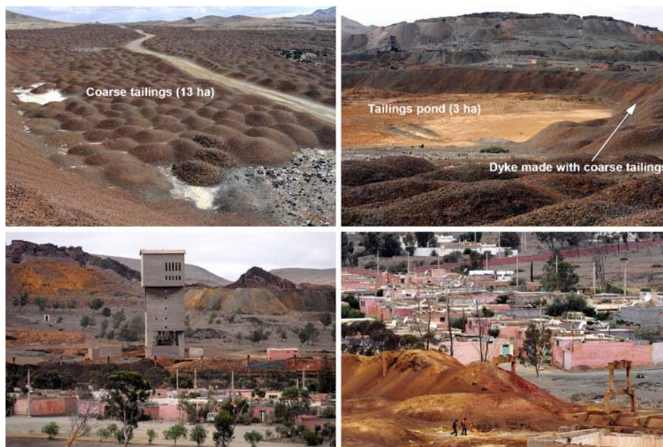
Fig. 2 Photographs illustrating the AMD problem at the Kettara mine site
